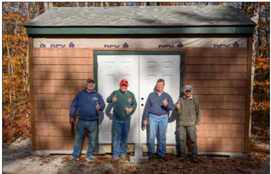
LPC extends its deepest gratitude to the Meredith Rotary Club Major Projects Committee for granting up to $20,000 to excavate an area near the Field Operations Center to construct a storage building to house equipment and supplies. The Club purchased the supplies and volunteers constructed the shed. Rotary Crew: Dan Whitney, John Columbus, Bruce Reichlen, and Ron Maher
