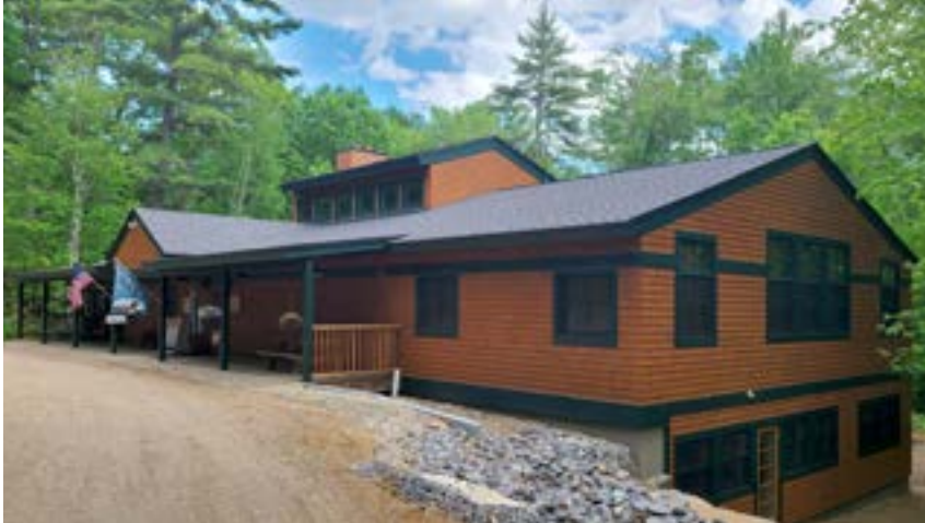
The expanded Loon Center includes new office and meeting spaces, an upgraded laboratory, and dedicated storage for field supplies and biological samples, including a walk-in freezer.
